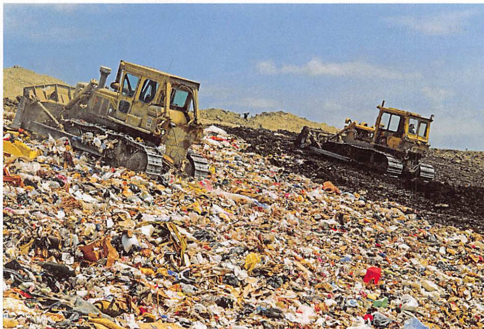
Figure 1.10 Sites such as this landfill are all-too-frequent reminders of the adverse environmental impacts of humans and their waste products. Here, bulldozers compact solid waste and spread a daily cover at a "sanitary" landfill.
