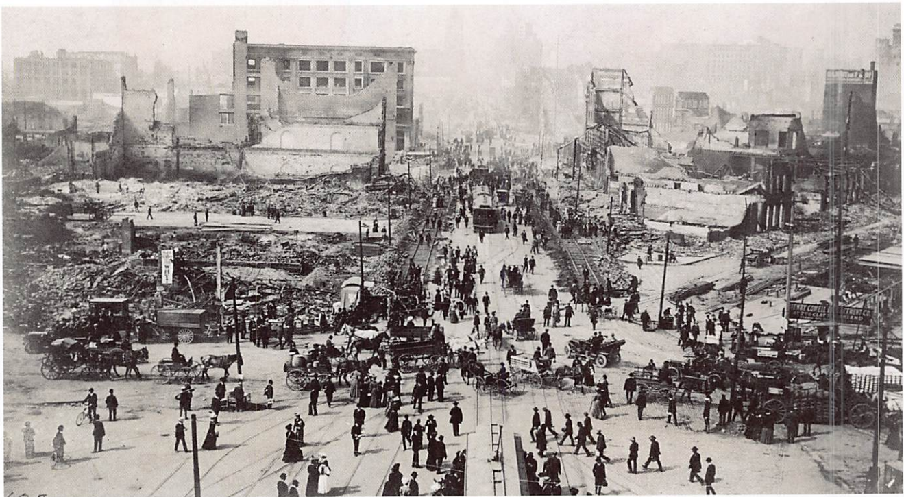
Figure 3.21 Destruction from the San Francisco earthquake and fire. The first shock struck San Francisco early on the morning of April 18, 1906, damaging the city’s water system. Fire broke out and raged for three days. It was finally stopped by dynamiting buildings in its path. When it was over, some 700 people were dead or missing, and 25,000 buildings had been destroyed. Locally, the event is usually referred to as the Great Fire of 1906, suggesting a denial of the natural hazard in favor of assigning blame to correctable human error. Post-destruction reconstruction began at once. Rebuilding following earthquake damage is the general rule.
