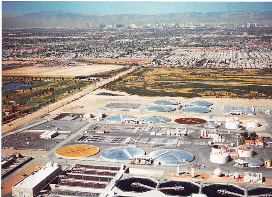
Figure 4.18 Pure piped water replacing individual or neighborhood wells, and sewers and waste treatment plants instead of privies, became increasingly common in urban Europe and North America during the 19th century. Their modern successors, such as the Las Vegas, Nevada, treatment plant shown here, helped complete the epidemiologic transition in developed countries. Lynn Betts, USDA, Natural Resources Conservation Center
