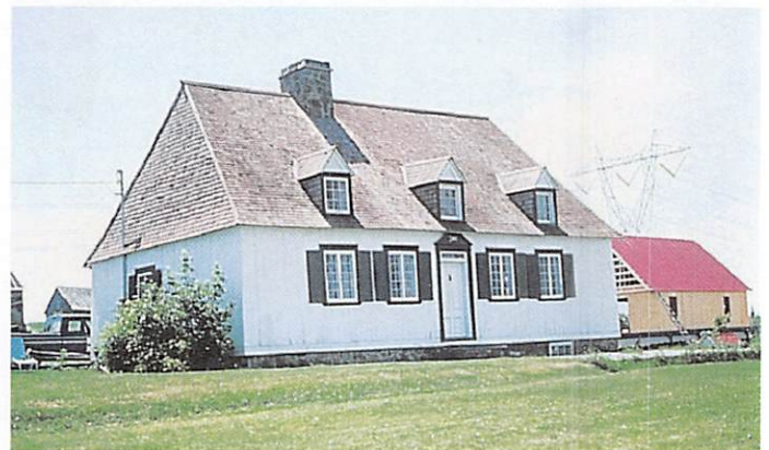
Figure 7.31 Vernacular house types in the Lower St. Lawrence hearth region of Quebec, Canada, included the Norman cottage with steeply pitched, hipped roofs and wide or upturned eaves, nearly identical to houses in the Normandy region of northern France.
