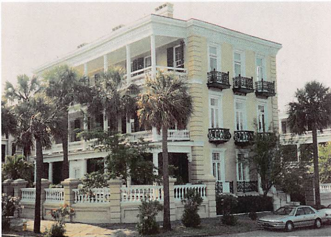
Figure 7.37 The Charleston single house of the Southern Tidewater hearth. The name refers to its single row of three or four rooms arranged from front to back and lined on the outside of each floor by a long veranda extending along one side of the structure. It resembles an I house turned on its side and shaded with a veranda from the hot southern sun.
