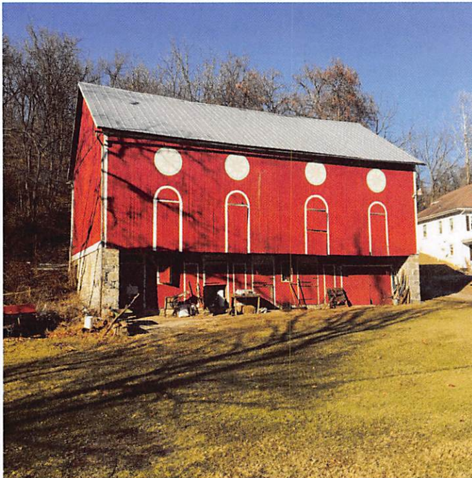
Figure 7.3 The Pennsylvania Dutch barn, with its origins in southern Germany, has two levels. Livestock occupy the ground level; on the upper level, reached by a gentle ramp, are the threshing floor, haylofts, and grain and equipment storage. A distinctive projecting forebay provides shelter for ground-level stock doors and unmistakably identifies the Pennsylvania Dutch barn. The style, particularly in its primitive log form, diffused from its eastern origins, underwent modification, and became a basic form in the Upland (i.e., off the Coastal Plain) South, Ohio, Indiana, Illinois, and Missouri. It is an example of a distinctive ethnic imprint on the landscape that became part of the material folk culture of the United States.
