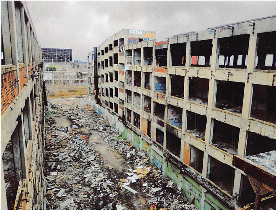
Figure 7.24 The direct landscape of the vacant Packard automobile manufacturing plant in Detroit, Michigan offers landscape evidence of the creative destruction of capitalism.
