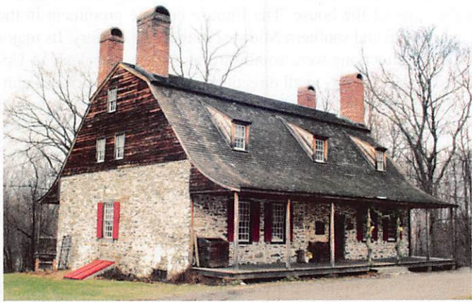
Figure 7.32 Dutch colonial houses, found in New York’s Hudson Valley, have a distinctive gambrel roof that gives more headroom in the top floor by using two slopes for the roof.
