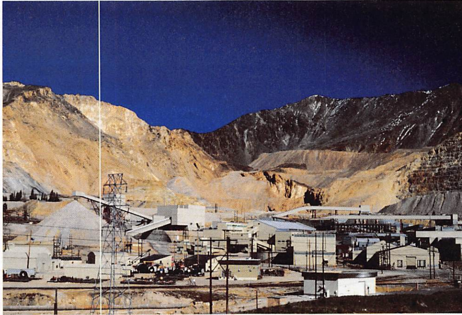
Figure 8.31 Molybdenum mine and concentrating mill at the open pit mine in Climax, Colorado. Concentrating mills crush the ore, separating molybdenum-bearing material from the rocky mass containing it. The great volume of waste removed ensures that most concentrating operations are found near the ore bodies. Because concentrating is a “weight-reducing” process, it saves transportation costs to locate it close to the mine.
