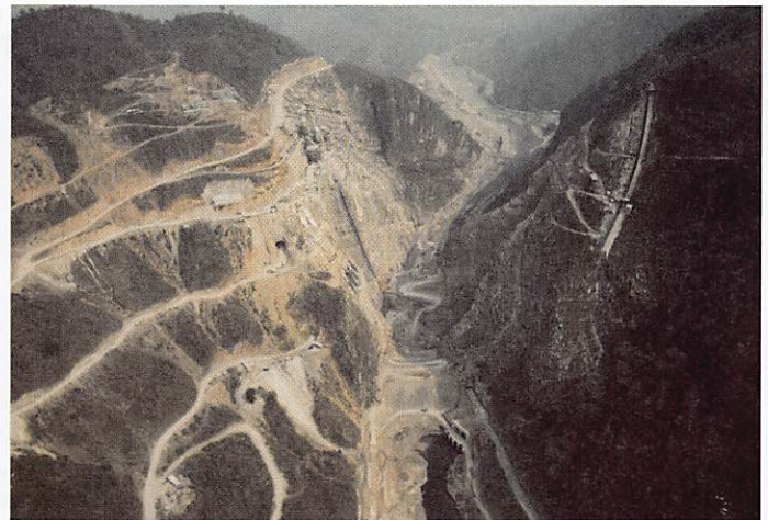
Figure 10.19 The El Cajón Dam in Honduras is an example of a technology transfer development project funded by the World Bank. Honduras lacks fossil fuel supplies but was felt to have a comparative advantage in hydroelectric power generation thanks to its rugged topography and powerful rivers. The 226-meter (741-foot)–high dam cost almost $800 million when it was built in the 1980s. The amount of debt required for the dam was staggering for a country with just 5 million residents and a per capita income of $590 per year in 1990. The dam failed to stimulate enough economic growth to pay back the loans and contributed to Honduras being classified by the IMF and World Bank as a HIPC. The electricity was delivered to the cities, where it was used by new, export-oriented textile industries. Meanwhile, many rural areas of the country still lack electricity, and peasant farmers living near the dam lost their livelihoods when their lands were flooded by the reservoir.
