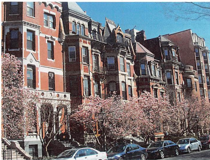
Figure 11.20 Townhouses, such as these in Boston’s Back Bay area, as well as apartment buildings and duplexes, were a characteristic response to the price and scarcity of developable urban land in the era before automobiles became widely available. Where detached single-family dwellings were built, they were typically on smaller lots than became the norm once widespread automobile use allowed cities to spread outward in the second half of the 20th century.
