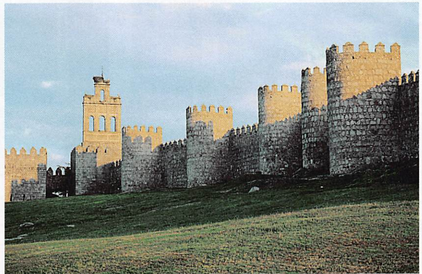
Figure 11.10 By Europe's Middle Ages, the ancient need for city protection remained, but fortifications and defensive structures had assumed elaborate and massive forms that were unknown and unneeded before siege weapons and siege warfare put all cities in jeopardy. The walls of Ávila, Spain, shown here, were built in the 12th century, extending 2,500 meters (8,200 feet) and encircling the entire city at that time; the modern part of Ávila lies outside.
