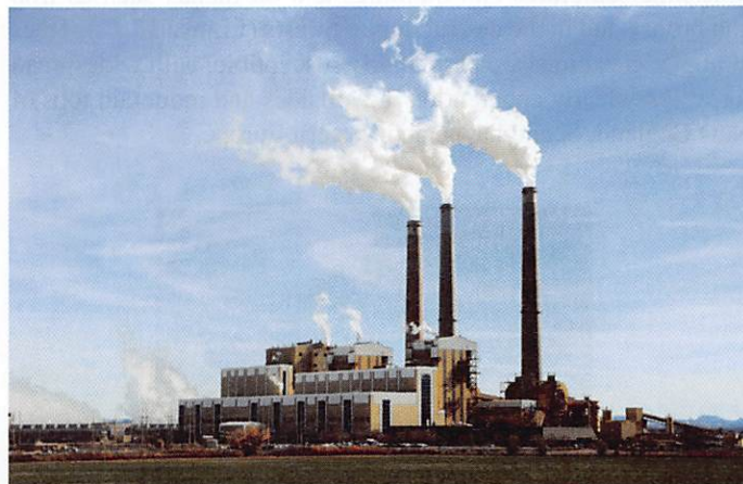
Figure 13.10 Dilution is not the solution to pollution. Before concern about acid rain became widespread, the U.S. Clean Air Act of 1970 set standards for ground-level air quality that could be met most easily by building tall smokestacks high enough to discharge pollutants into the upper atmosphere. Stacks 300 meters (1,000 feet) and higher became common at utility plants and factories, far exceeding the earlier norm of 60–90 meters (200–300 feet). What helped cleanse one area of pollution greatly increased damage elsewhere.
