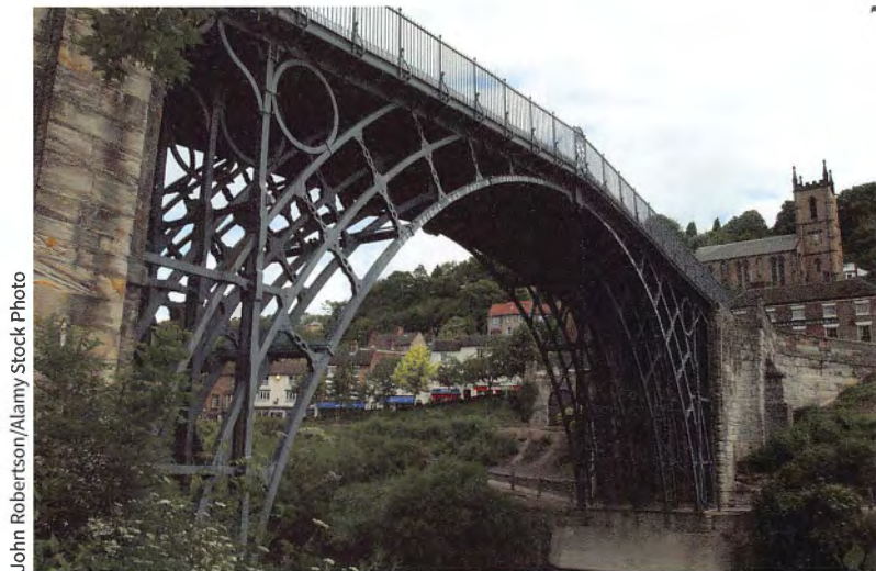
FIGURE 12.3 Ironbridge, England. The world’s first bridge made entirely of cast iron was constructed in the late eighteenth century near Coalbrookdale, England, reflecting the resources, technology, and available skills in this area at the time.
